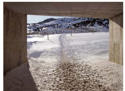
View, facing west, of the deer trail through the underpass.
