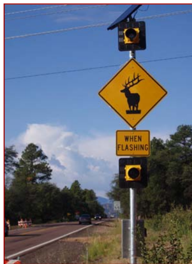
Figure 4.5. Array of signs presented to motorists as they approach the SR 260 wildlife crosswalk. A static sign (top) alerts motorists that the detection area lies ahead, while the variable message board (middle) and the flashing lights on the elk silhouette sign (bottom) are only activated when animals were detected by the RADS.
