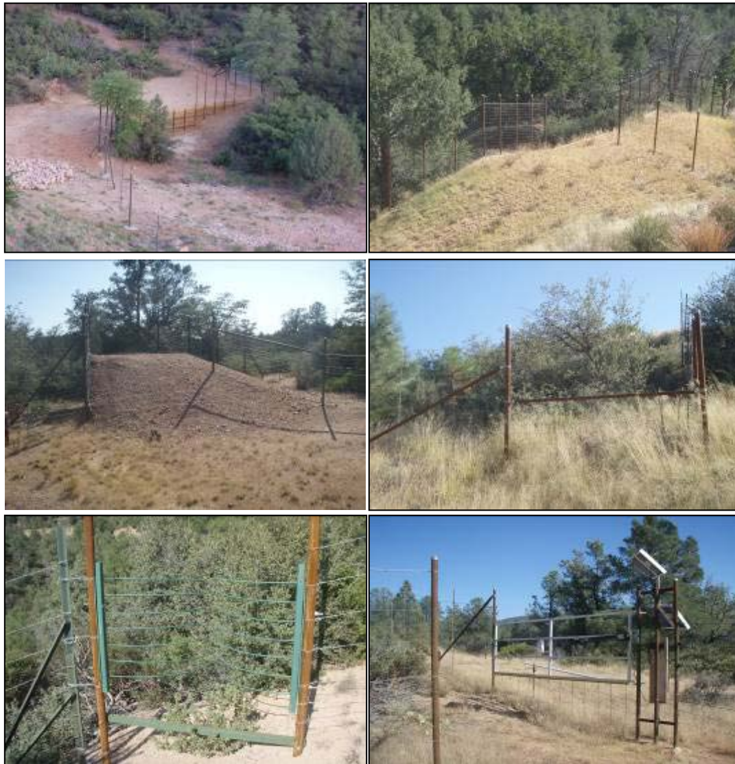
Figure 4.2. Right-of-way wildlife escape mechanisms incorporated into the project in the event elk entered the ungulate-proof fenced right-of-way along the Preacher Canyon section, State Route 260, Arizona. These mechanisms include three engineered escape ramps (top two and middle left photos), “slope jumps” installed in corners of the fencing (middle right photo), one-way gates (bottom left photo) and a pair of animal-activated electric gates (bottom right).
