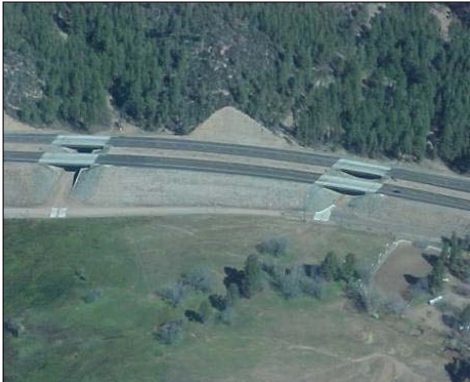
Figure 3.3. Aerial photographs of the Preacher Canyon Bridge (top) and the west and east underpasses at Little Green Valley along the PC section.
