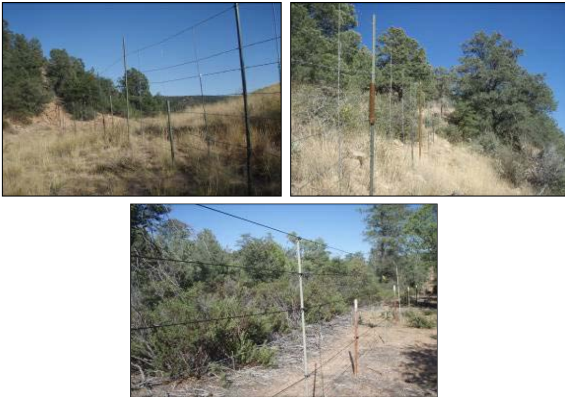
Figure 4.1. Types of retrofit fencing used to funnel animals to existing passage structures and the crosswalk along SR 260, including 10-ft T-posts and barbed-wire (top left), T-post sleeve extensions and barbed-wire (top right), and ElectroBraid™ electric fence modifications to extend the existing ROW fence to 7.5–8 ft.
