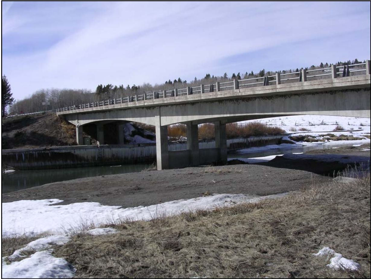
Photo 1. Buffalo Fork bridge (view northwest).
