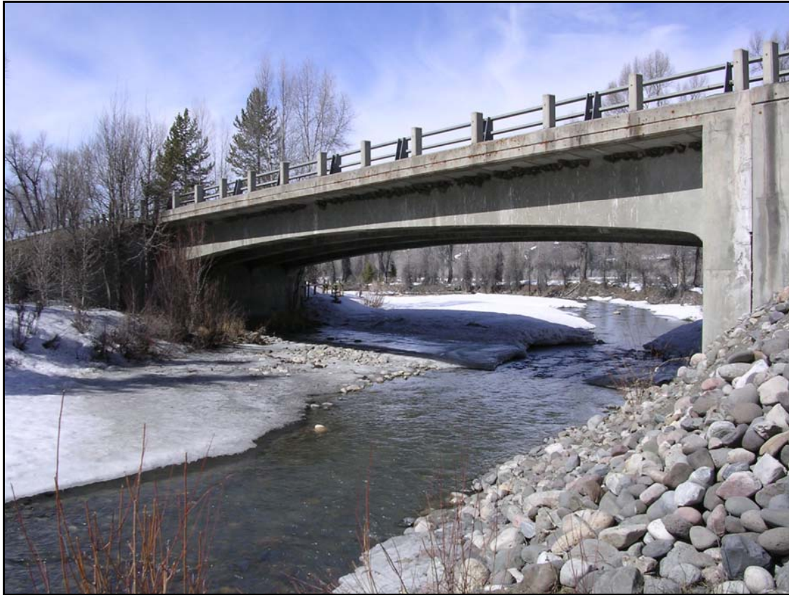
Photo 3. Blackrock Creek bridge (view north).
