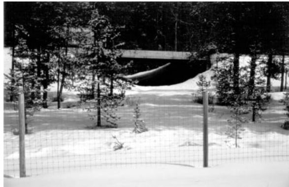
Highway mitigation fencing and wildlife underpass in Banff National Park, Alberta.
